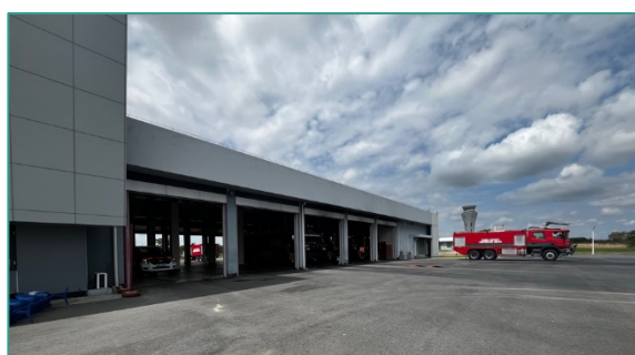
New Emergency Control Centre
