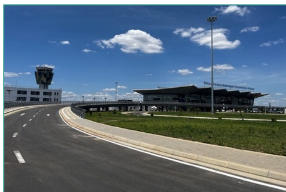
Vehicle access ramp
