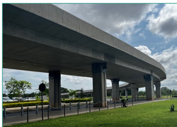
Vehicle access ramp
